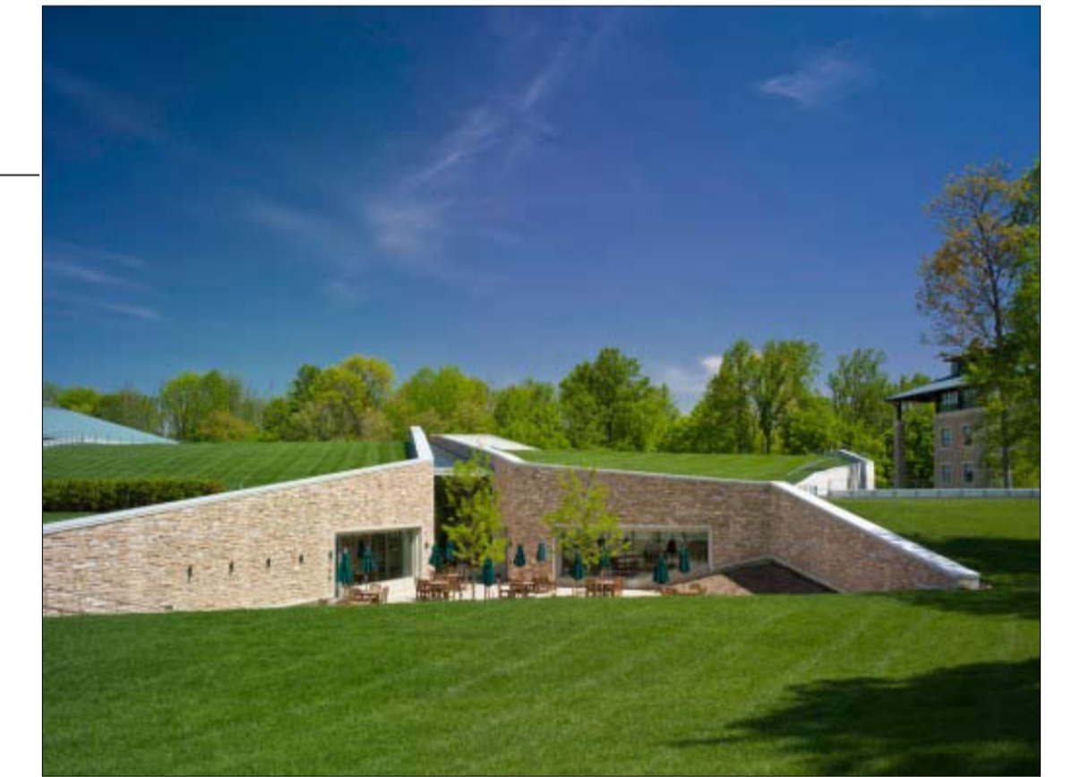
Becton Dickinson Campus, Franklin Lakes, USA
